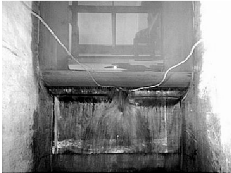
Figure 8. Ogee ventilated by means of hoses.
