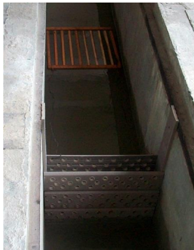
Figure 4. Soothing of flow waters under the discharge of the seating capacity weir.
