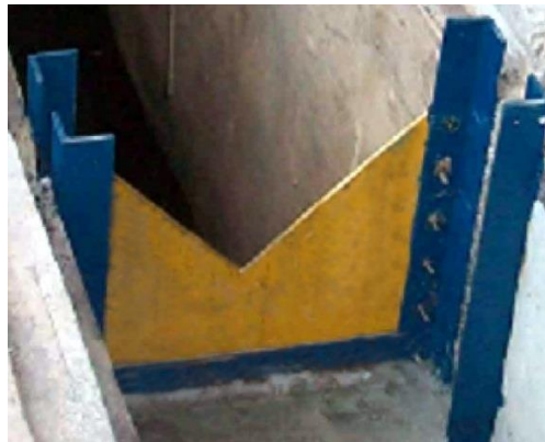
Figure 3. Seating capacity weir seen from downstream.
