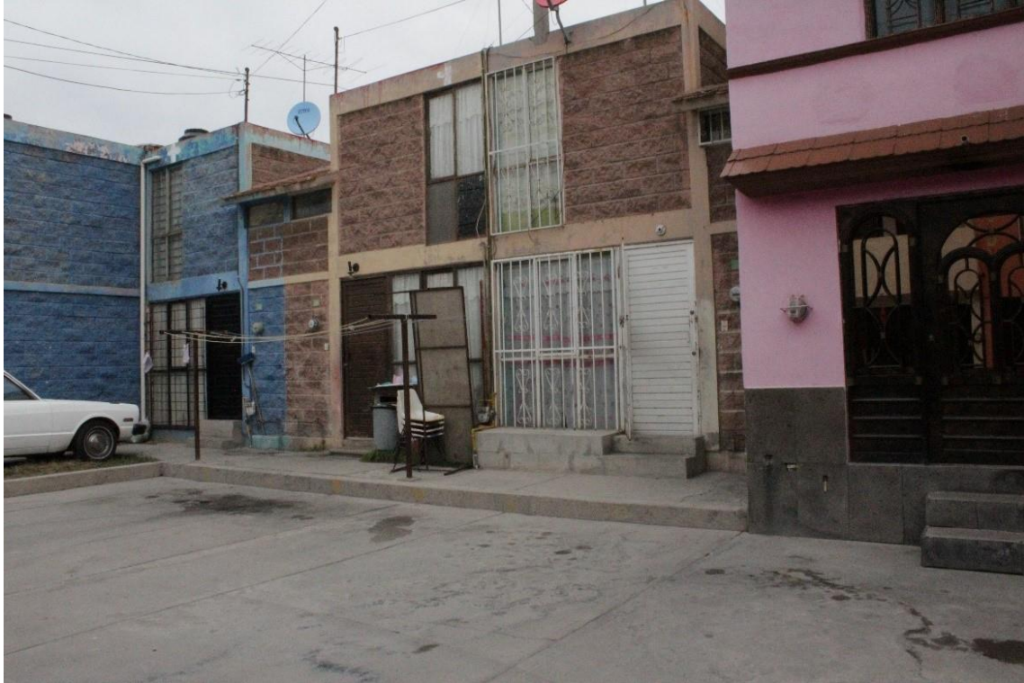
Figure 10. House modifications prevent rainwater from entering the houses (source: fieldwork 2018).
