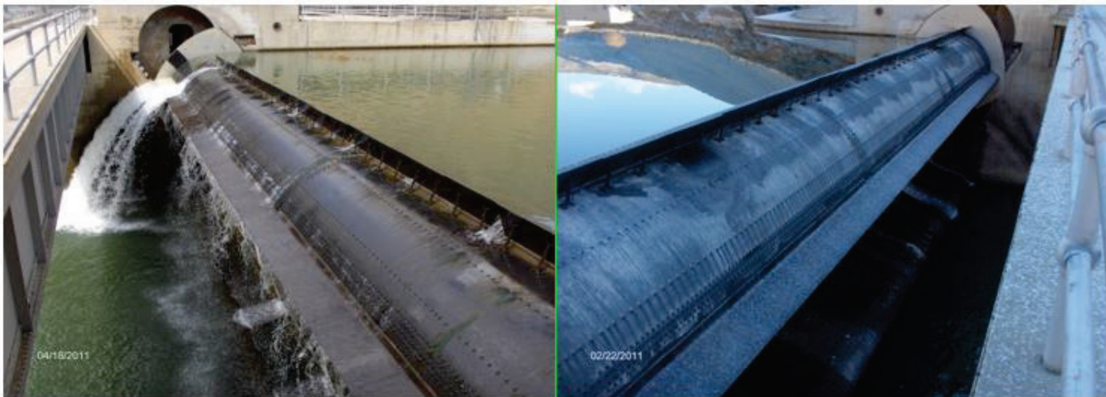
Figure 1. Roller Spillway at Roza Dam, United States. Source: USBR, 2010.
